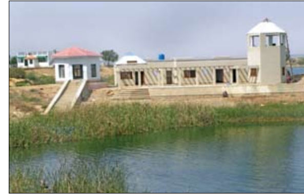
■ Keenjhar Conservation & Information Centre, construction work in final stages
